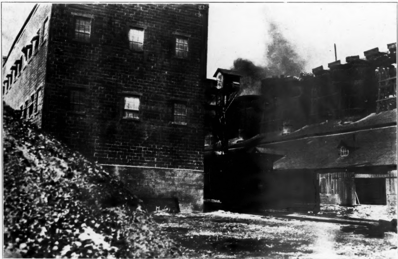
The Hydrate Building at Left and the Kiln at Right. Note the String of Cars Being Discharged Into the Top of the Kiln. Little Smoke is in Evidence Indicating Efficient Burning.
